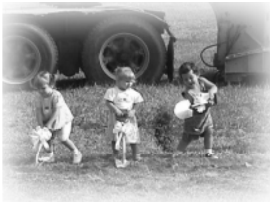
Weren't these kids having fun at the OCC child care center groundbreaking?
