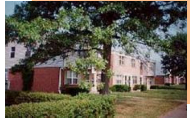
The Lincolnshire/Lincolnshire North Apartment Complexes
